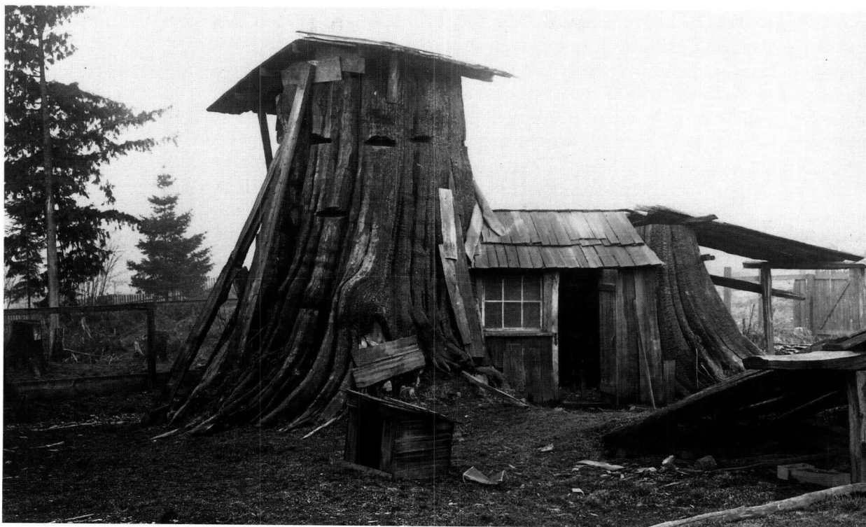
Mount Pleasant pioneer's shack in stump. It was built by a Mr. Berkman, and was on the east side of Seacombe Road, now Prince Edward Street, between 26th and 27th Ave. It was reached by a short forest trail from Horne Road, now 28th Avenue. The lower stump on the right was the kitchen, and the lower part of the higher stump on the left was the livingroom. The bedroom, doorless, was in the top of the higher stump and was reached by a ladder removed in daytime to the kitchen. According to Major J.S. Matthews, this photo was taken before 1910 by W.J. Moore, who lived nearby, and who also provided the particulars. cva Bu. P. 6, N. 31 #1.
