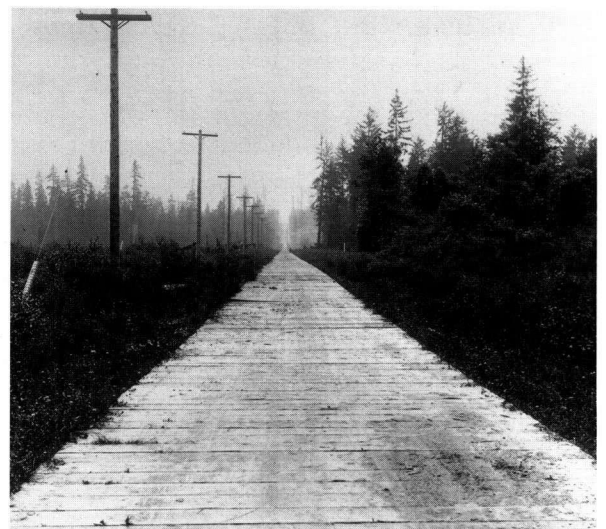
Kaye Rd., 1912, now Trafalgar St., looking south from 18th Ave. west. This area was so wet that it was better and cheaper to plank the muskeg rather than gravel it, as the gravel would sink out of site. CVA Str. P. 207, N. 149.
