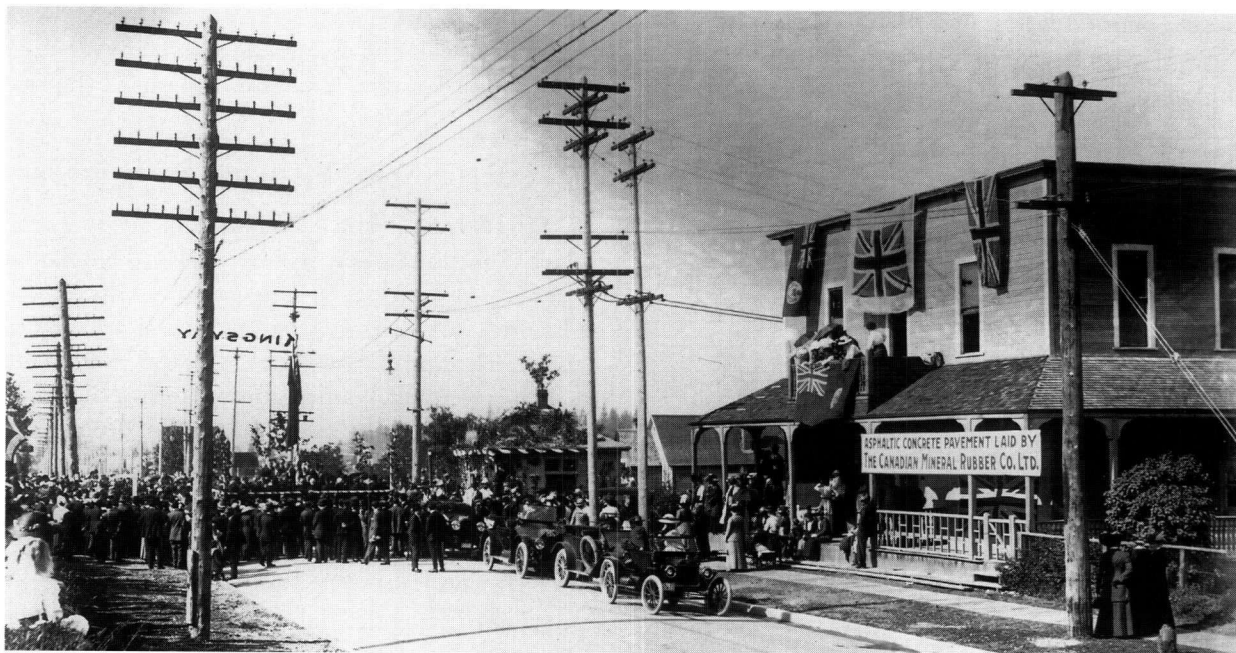
The opening of Kingsway, 30 September 1913, at Boundary Road by the Hon. Thomas Taylor, MLA, Minister of Public Works, Victoria. The open top automobile did not become unfashionable for several years. Speed limits must not exceed 25 miles per hour. A civic holiday in Burnaby, six hundred automobiles made the trip between New Westminister and Vancouver on the day the road was opened. CVA Str. P. 288. N. 338.
